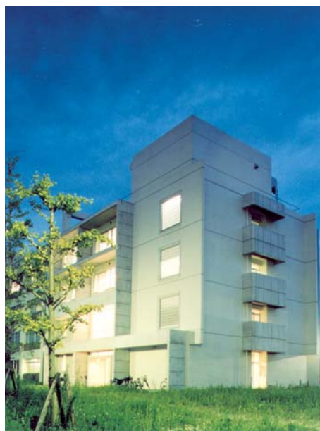
建物外観 Exterior View
