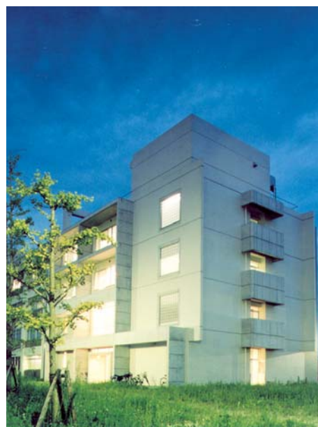
建物外観 Exterior View
